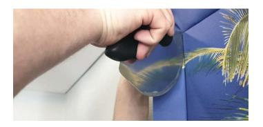
A harpoonless system whereby the textile is installed directly into a PVC wall profile or PVC ceiling profile.
