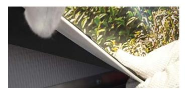
A system whereby the textile is lined with a PVC harpoon and installed in wall, ceiling or self-supporting aluminium profiles from the DPS Wall2Wall collection.
